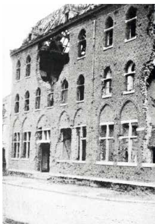
Little Talbot House in kantschool Lamotten
