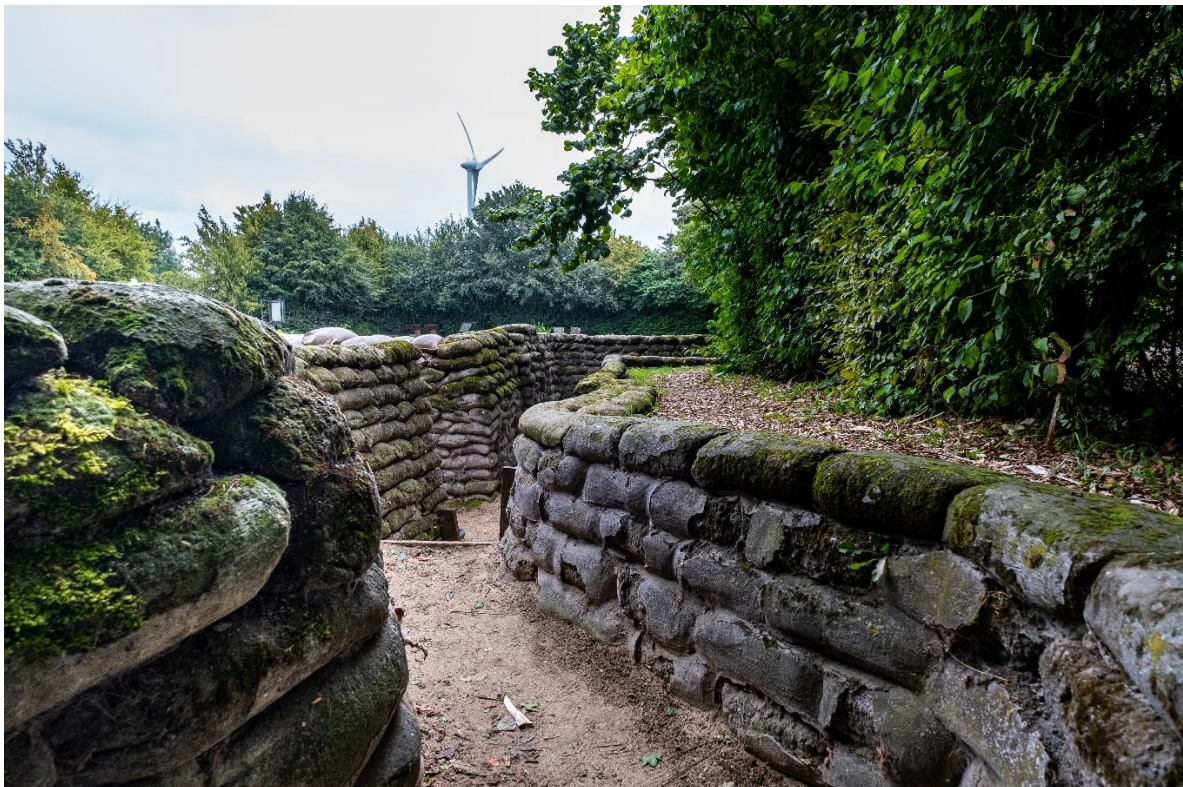
Photo 12 - Continued action remains necessary. Crumbling sandbags limit access to the trench.
