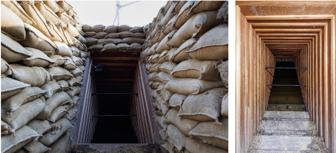
Photo 6 & 7 - The wooden stairwells, which give access to the dugout, have been renewed and the concrete nets have been replaced with black bars to allow visitors to safely glance into the dugout. Better lighting has also been installed. © Birger Stichelbaut
