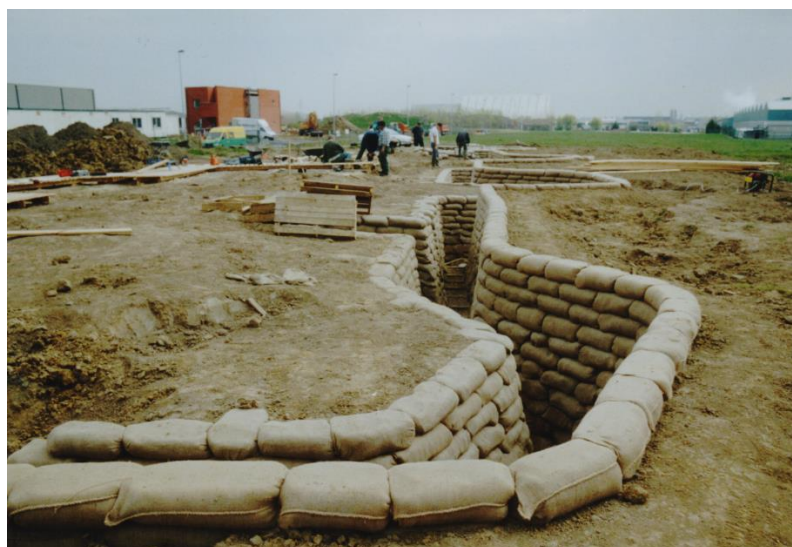
Photo 5 - The initial set-up of the site by The Diggers in 2002. © Patrick Van Wanzeele
